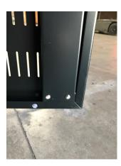
Remove the cover exposing the the lock and rod assembly. Grab the bottom of the cover and pull out and downward to release the cover from the door being careful not to bend the cover plate
