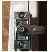
Step 4 - Place the locking tab (your tab may vary) so that it is 90 degrees from the lock assembly as shown and re-insert the flange bolt and tighten.
